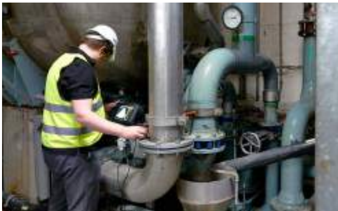
Industrial pipeline inspection with Proceq Flow Detector 100
