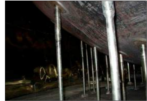
Bottom mounted instruments present a challenge for mechanical Integrity assessment
