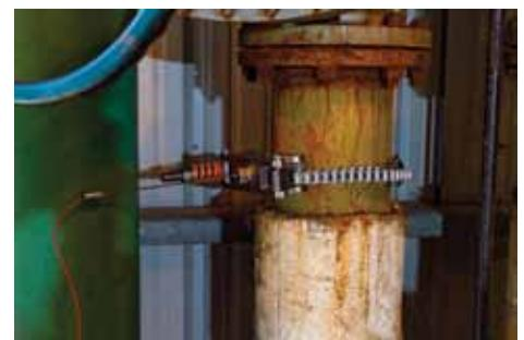
Rightrax™ permanently-installed sensor on oil & gas pipe section
