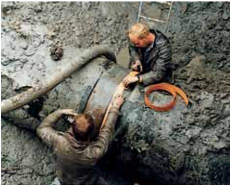
Oil & gas weld inspection using film
