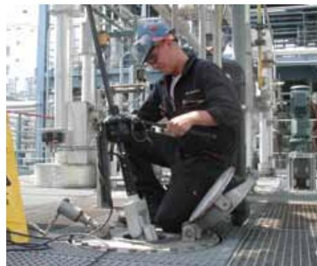
Inspecting chemical plant vessel with Ca-Zoom® PTZ inspection system
