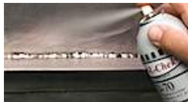
Typical aerosol application of D-70 during a weld inspection.
