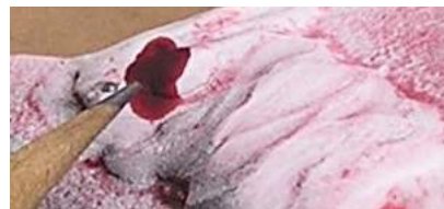
Visible Penetrant Indication on Weld
